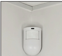
Installation to angle taking advantage of the base of the DG12 conceived for this type of solution, without need of I unwind
